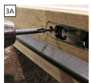
B. Insert the replacement rod into the top of the astragal. Twist to thread the rod into the mechanism.
