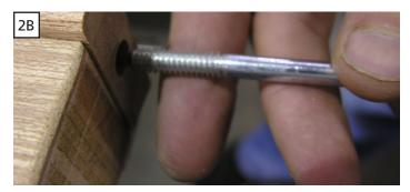
C. To remove the upper flushbolt mechanism, remove the attachment screws and remove the mechanism from the flushbolt rout.
