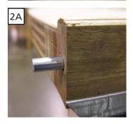
B. The top portion of the upper flushbolt is threaded into the flushbolt mechanism. Grasp the extended portion of upper flushbolt and twist to unthread and remove the upper flushbolt.
